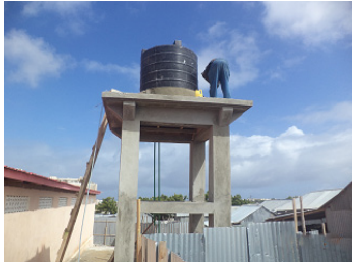
Top: Installing the solar pump for Sinay Market hall; the new water tank; the solid waste transfer station under construction. Bottom: The solid waste transfer station at different stages of construction.
